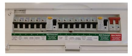
The label beneath the tripped switch will indicate which electrical system is tripping the electrics. This will help identify what is tripping the electrics and what not to use until the problem has been resolved.
